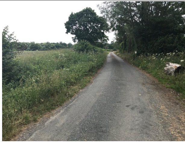
Verges along Ridley Hall Road G2
